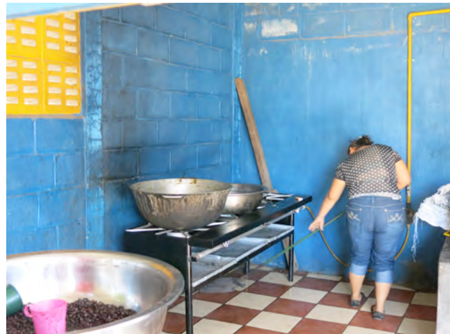
Renovation of propane fueled kitchen and delivery of propane.
